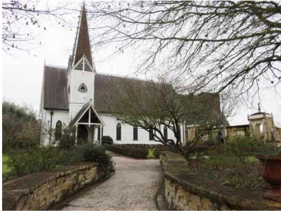
The Edythe Bates Old Chapel, built in 1883 and formerly the Travis Street United Methodist Church in La Grange, 16 miles away, was moved to the Round Top campus in 1994.
